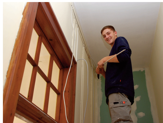
Installing electrical wiring at St. Rupert
