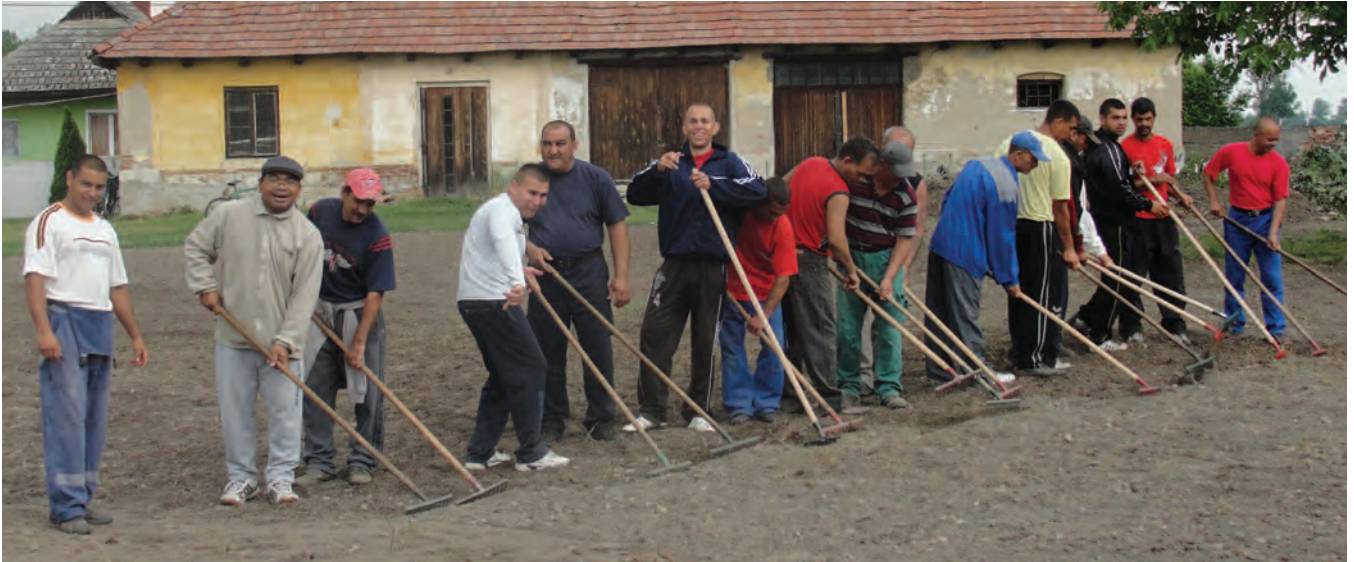
Work begins on the Blessed Ceferino Community Center.
