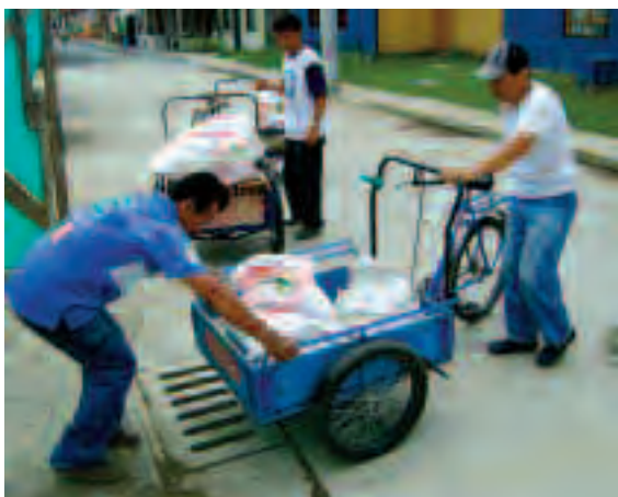
Bringing building material donated for construction
